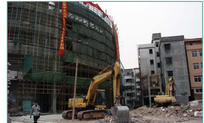
New wholesale mall under construction in GZ Drapery District (2007)
