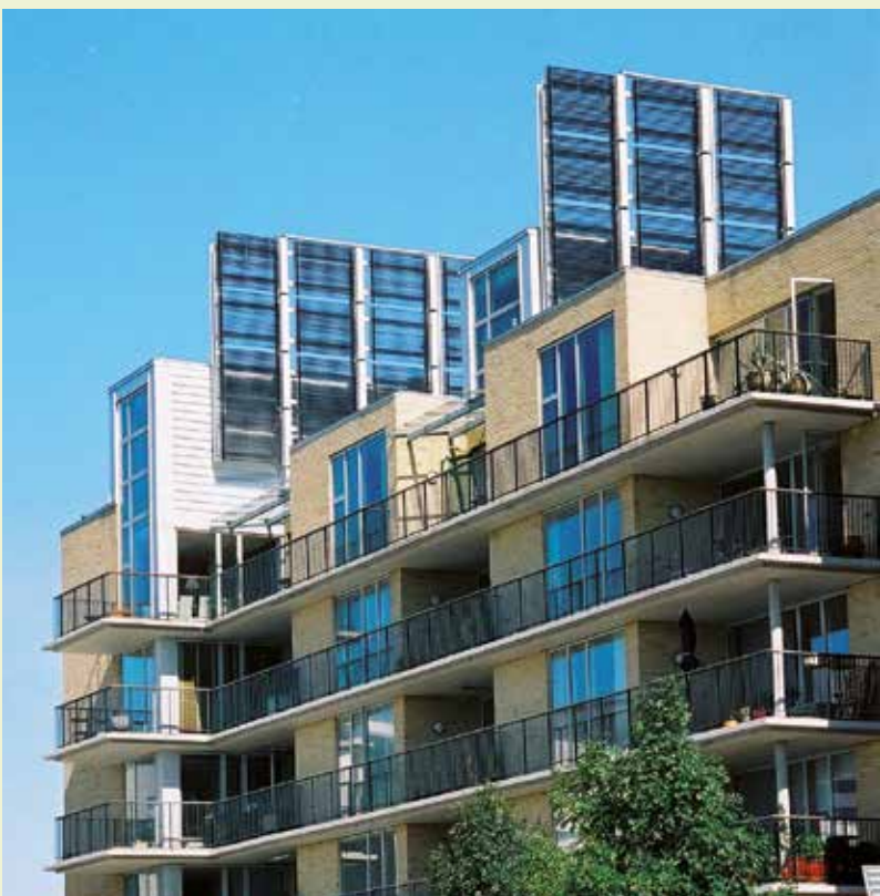
Solar thermal vacuum pipe collectors (fig. 4)
