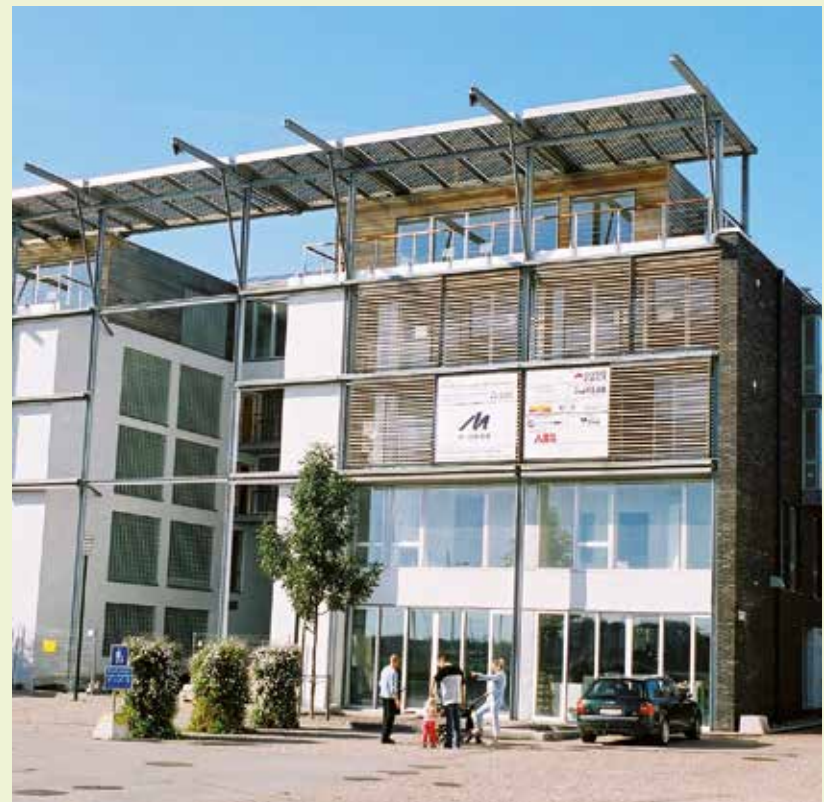
Protecting PV structure (fig. 5)
