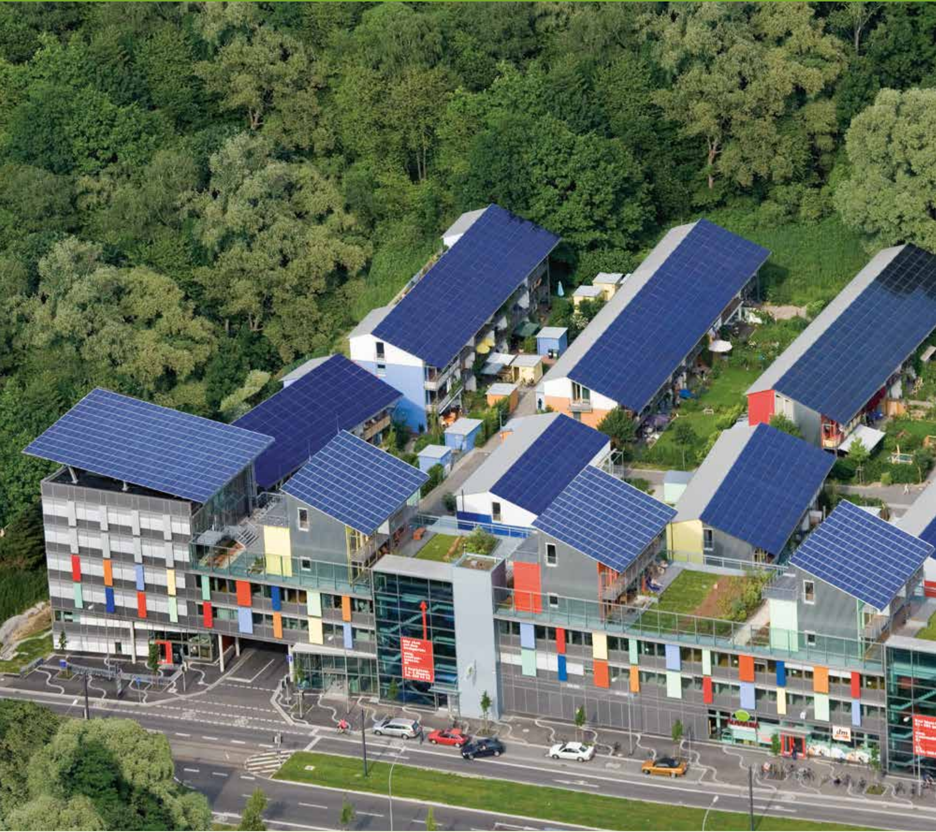
Solar Settlement with maximised PV roofs and passive-house energy standard (fig. 11)
