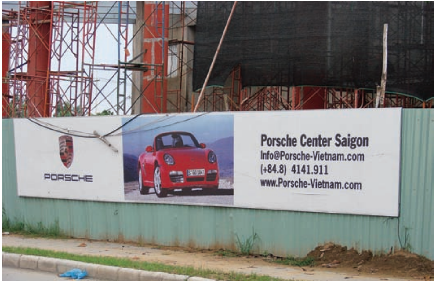
Photo 5: Showroom for the luxury car brand Porsche under construction in Saigon South
